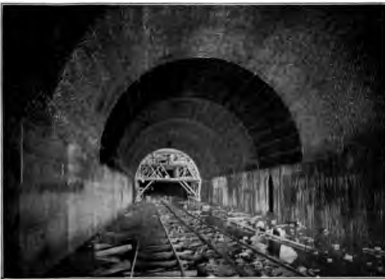
FINISHING THE LINING OF A TUNNEL
